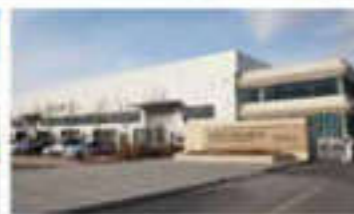
征和发动机链系统工厂 Engine Chain System Factory
